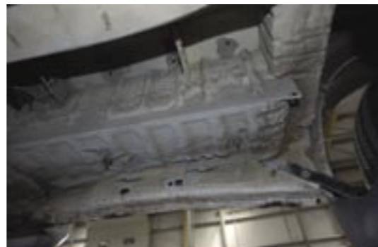
This underseal was factory applied by Ford; note all the bits that have been missed. It would be a similar story if this were any other brand of base vehicle – they all have pretty rudimentary rust-proofing as standard
